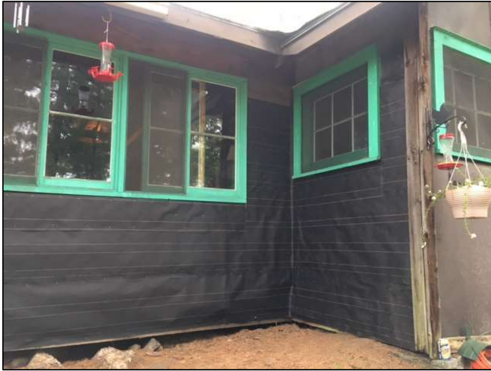
Tar paper replaced after siding was installed. This area will have exterior siding.
