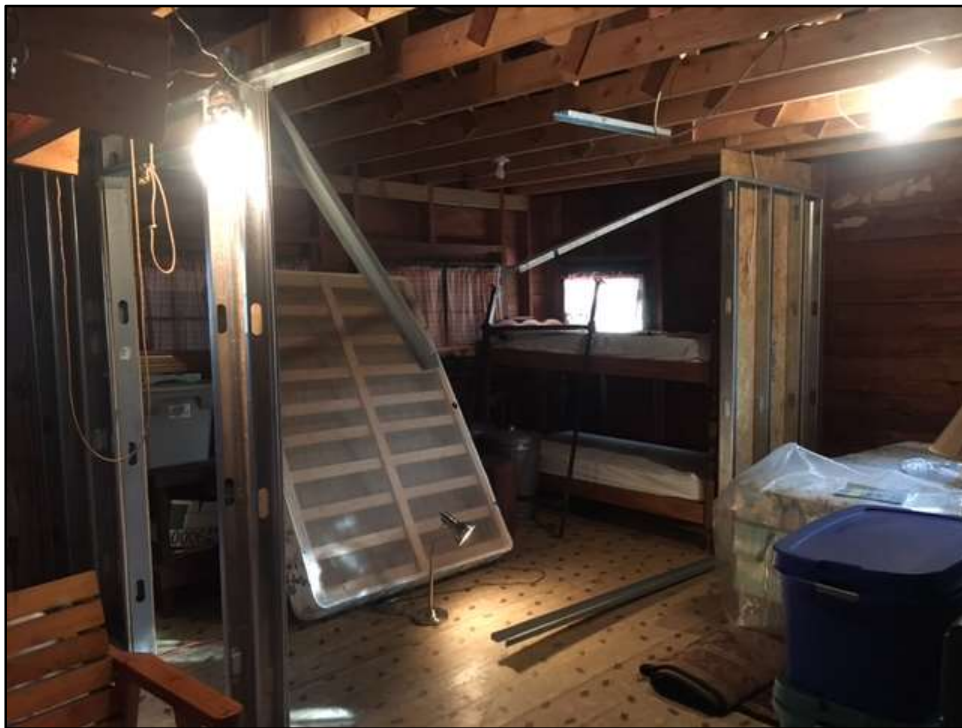
Partitions in the process of being removed from BH living room.
