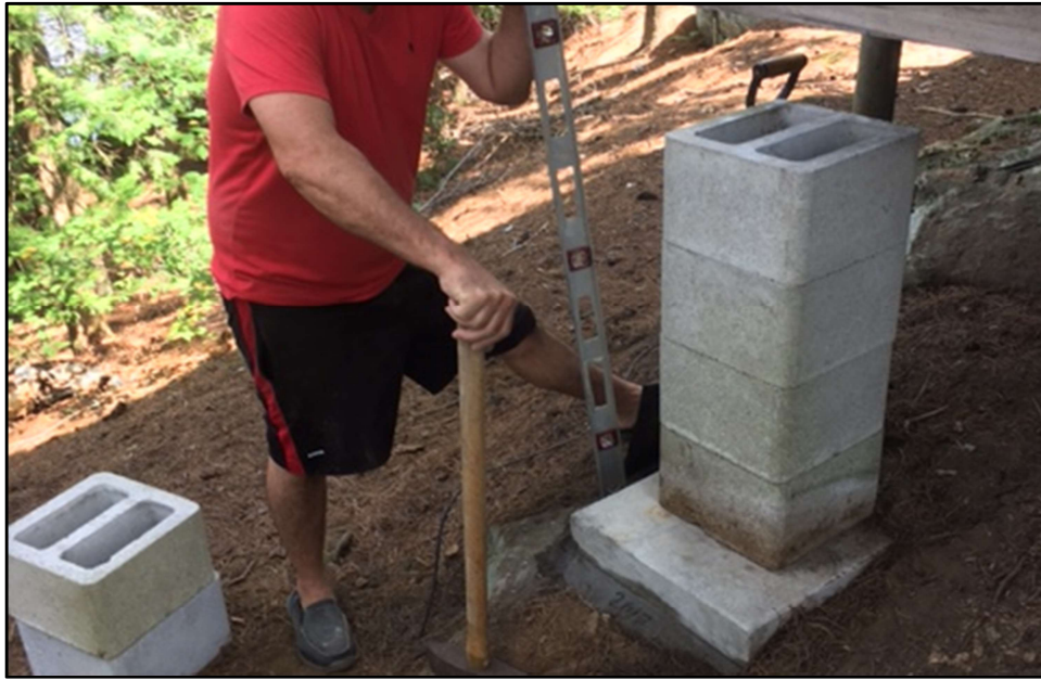
Cement pads and cinder block installation under BH kitchen.
