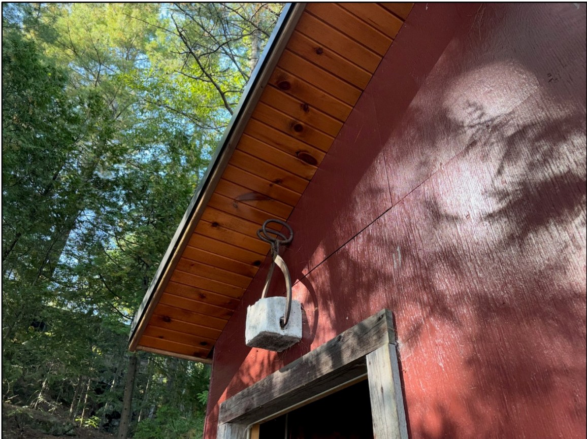
Overhead detail using knotty pine tongue and groove.
