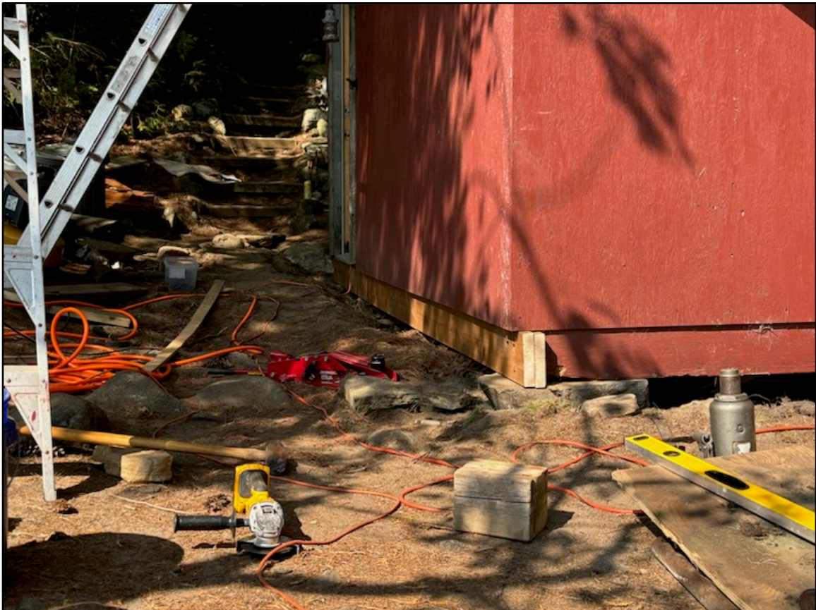
New treated lumber front beam.
