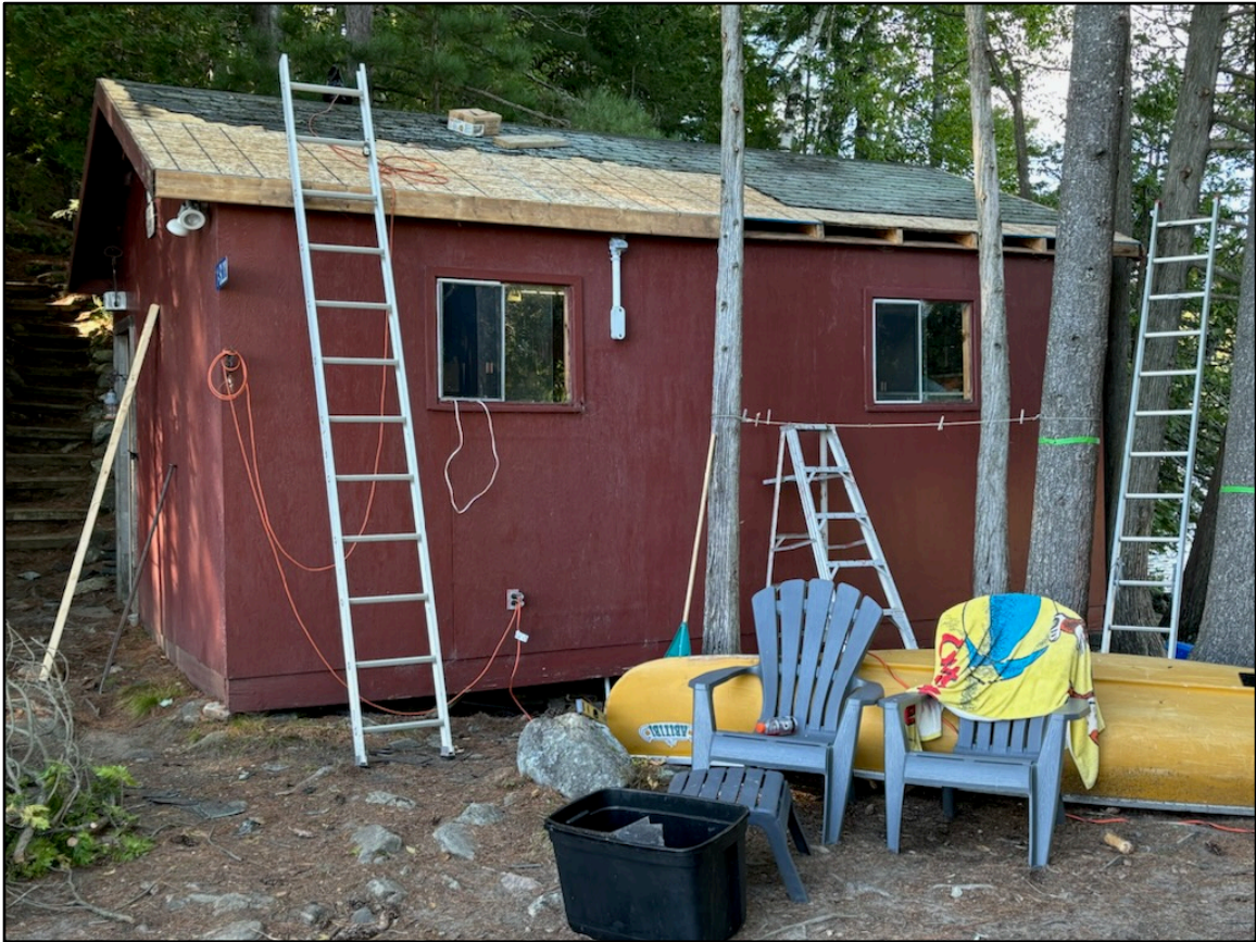
New roof sheathing and fascia boards being installed.
