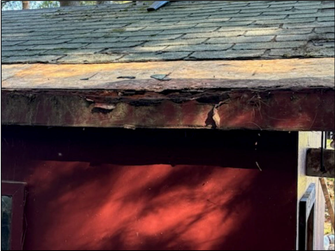
Rotted fascia boards and OSB roof sheathing.
