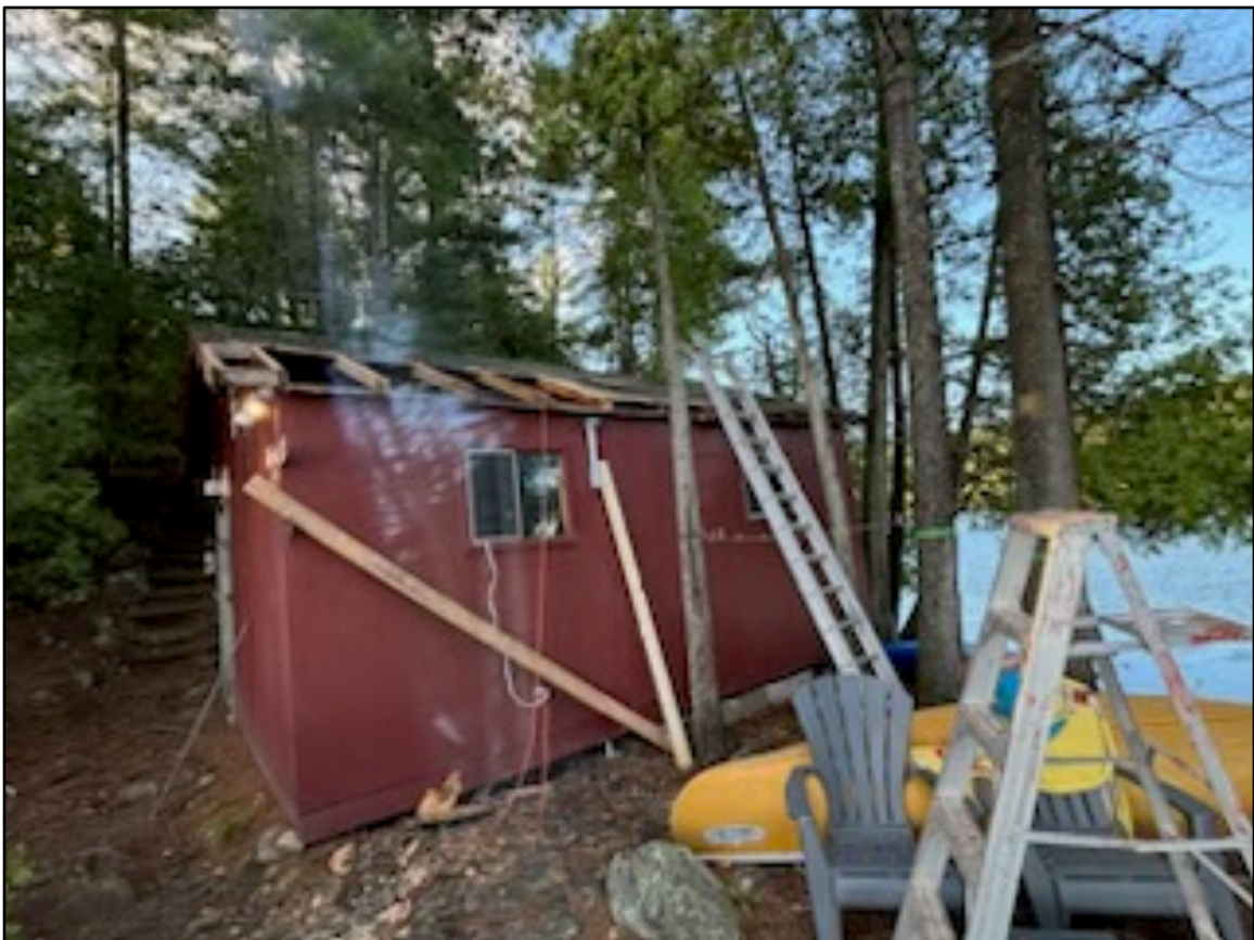
All fascia boards removed along with rotten sheathing.
