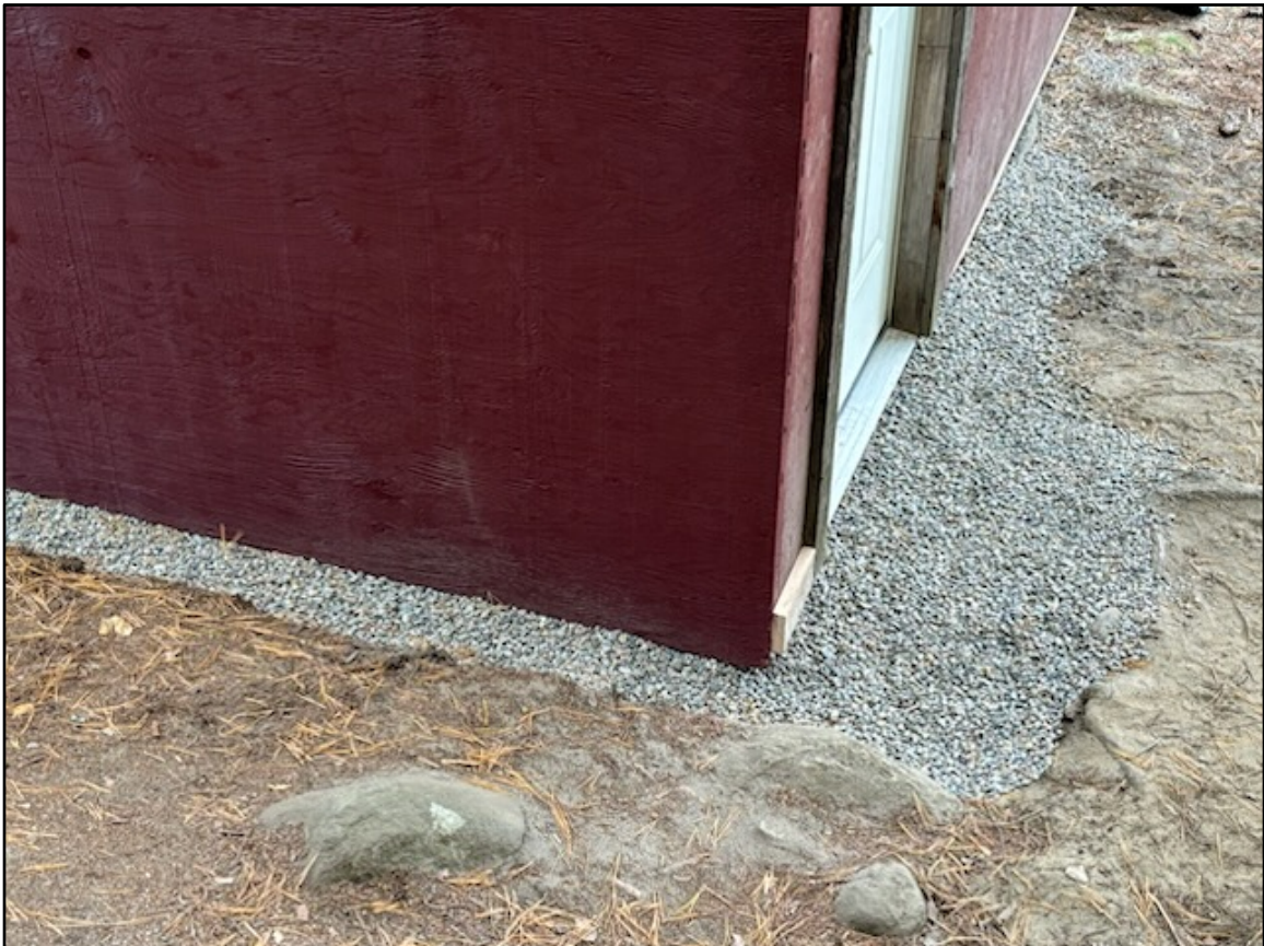
1 ton of quartz/granite gravel applied under floor.
