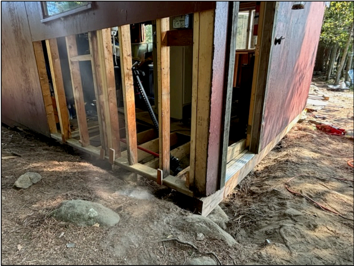
Siding and frame rot and repair.
