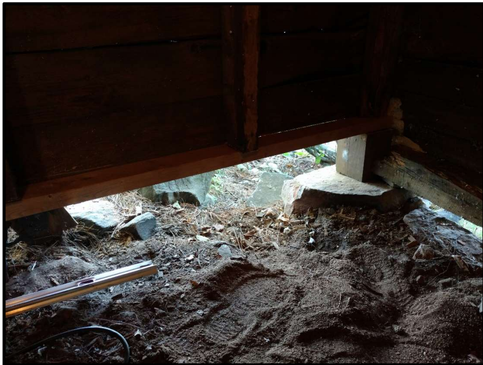
The reconditioned corner prior to adding a support beam and the cement foundation.
