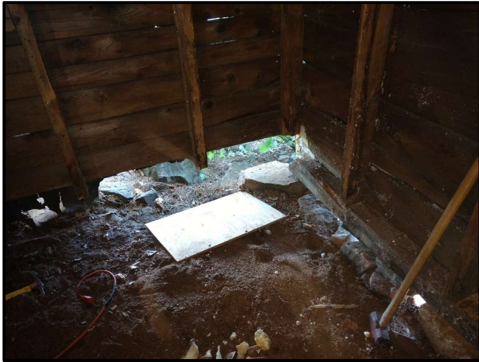
Rotted corner of guest house. This picture was taken after cutting out the affected wood and support beam.
