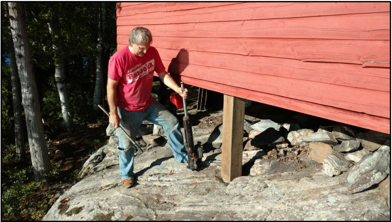
Little House porch leveling.
