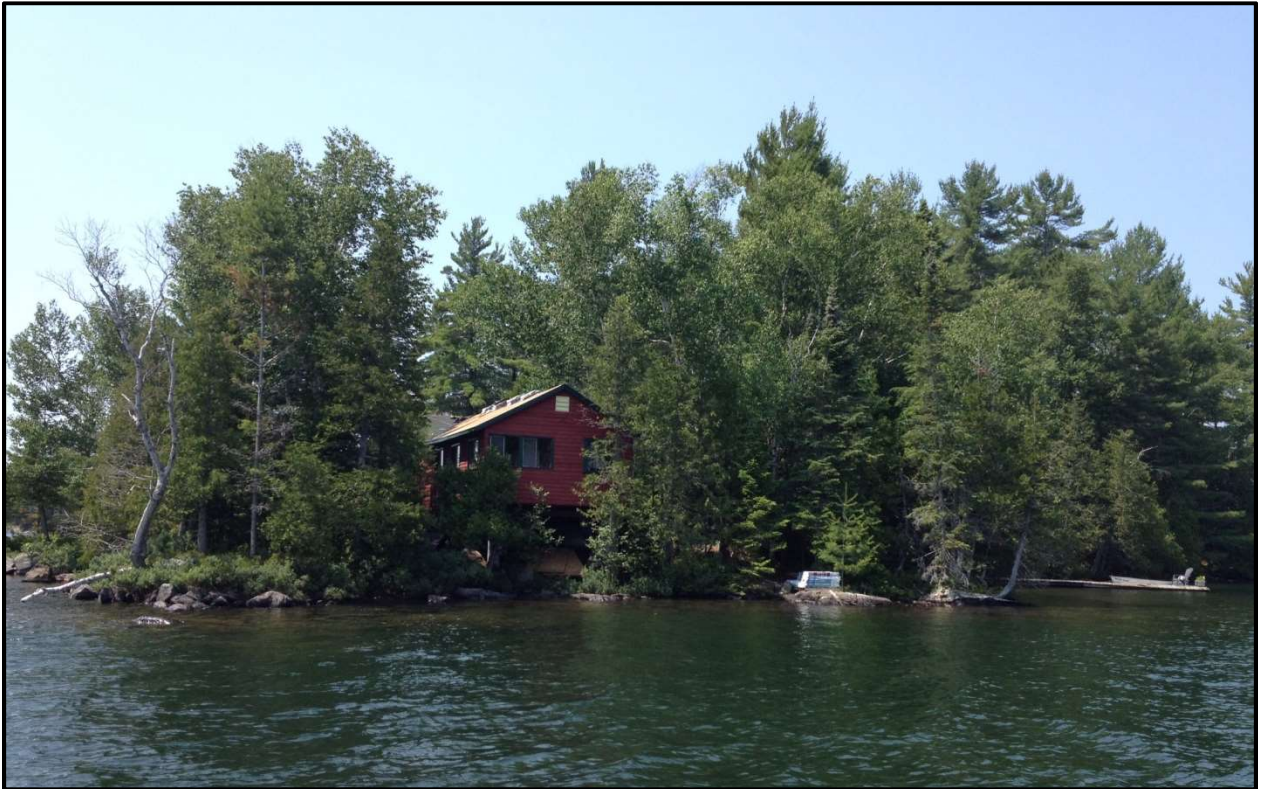
2015 Little House roof replacement.
