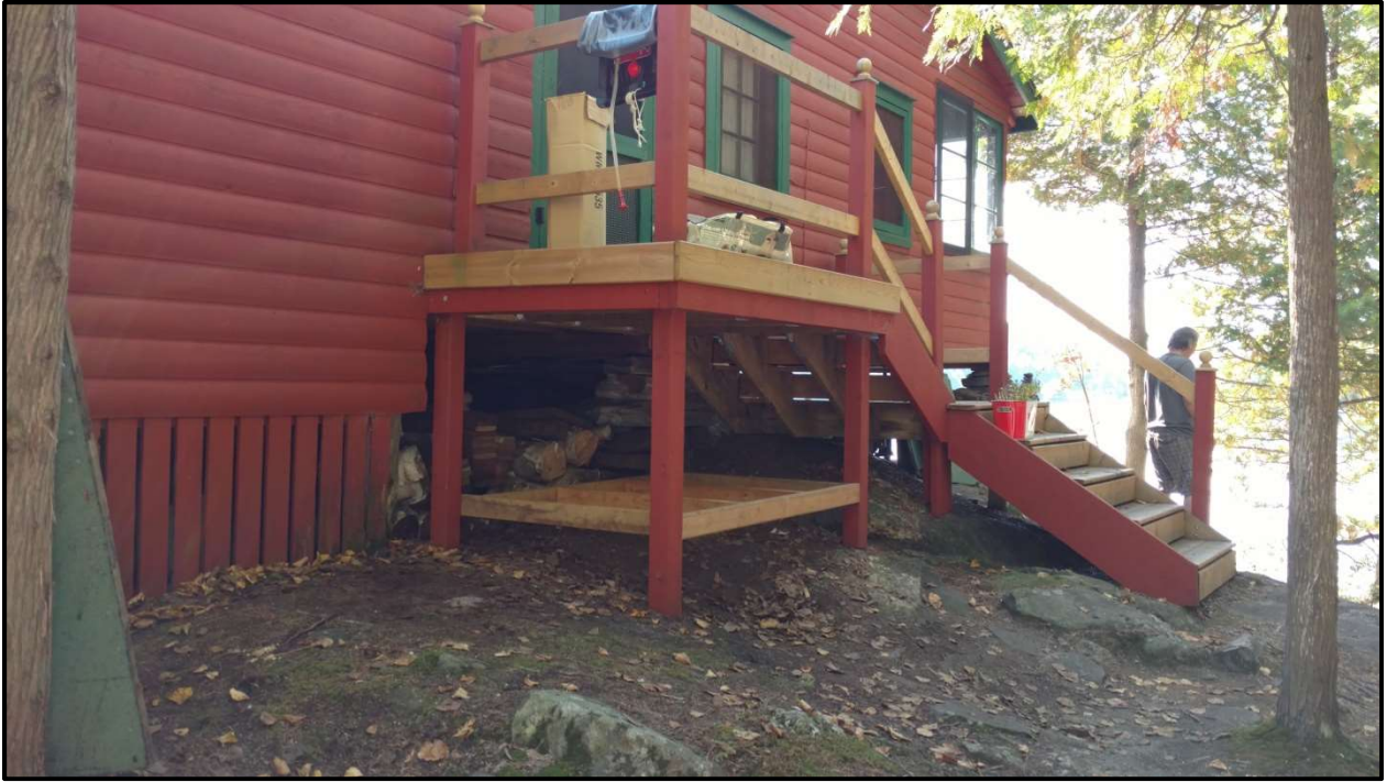
Lower railing and platform under stairs.
