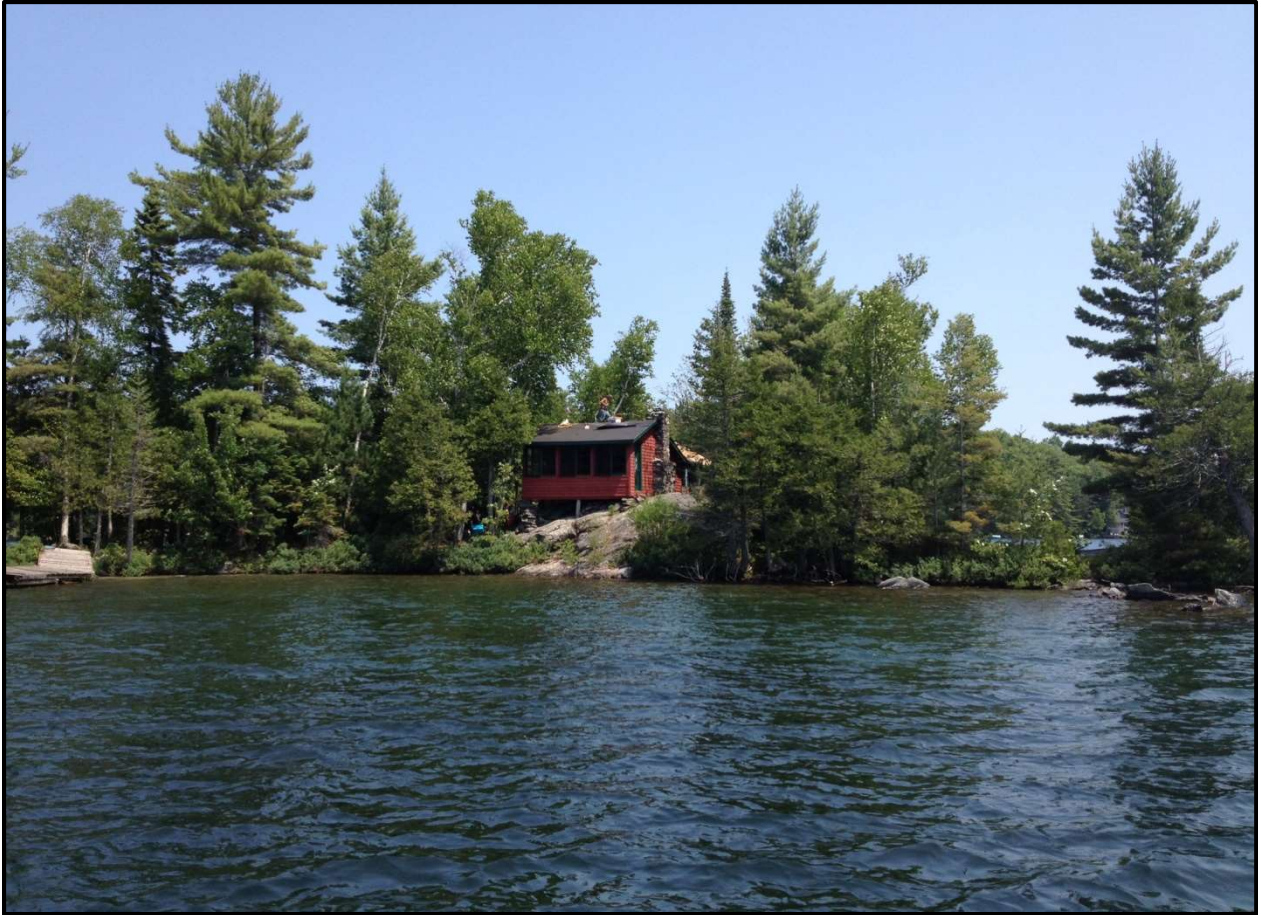
2015 Little House roof replacement.
