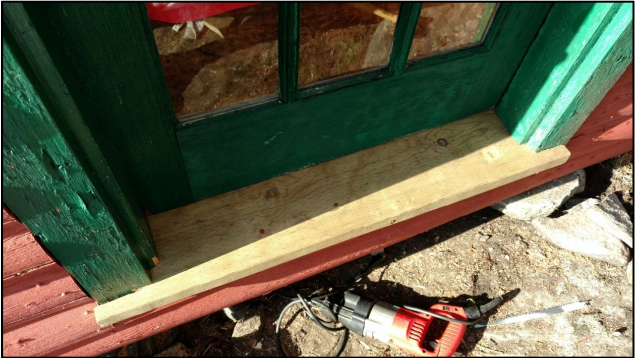
Little House porch door sill replacement.
